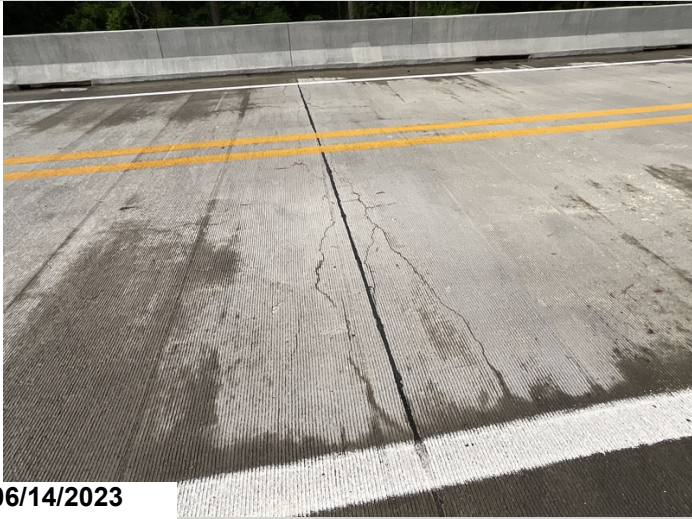
Deck cracks at bent 3 joint
