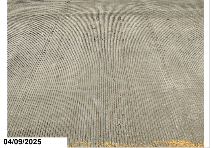
East approach slab cracking 24' CS2
